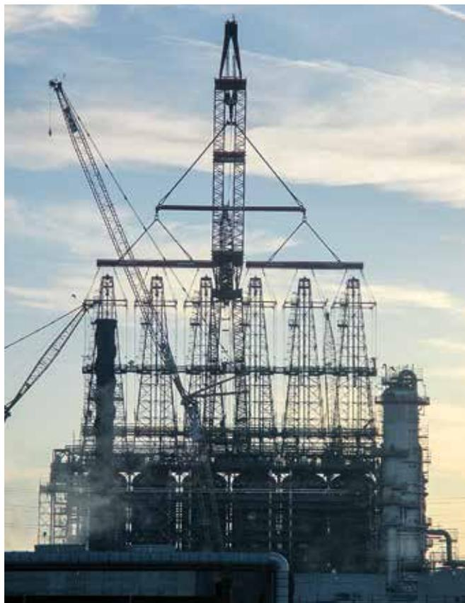
FIG. 3. The El Segundo project was an unique six-drum lift.
