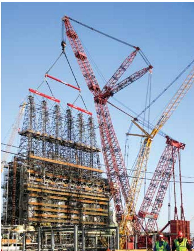
FIG. 2. Cranes and rigging in place for the main lift.
