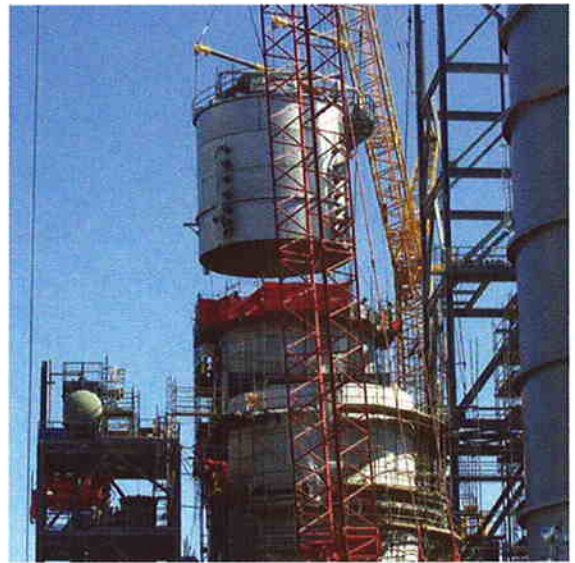
Nooter Construction project team erects new scrubber.
