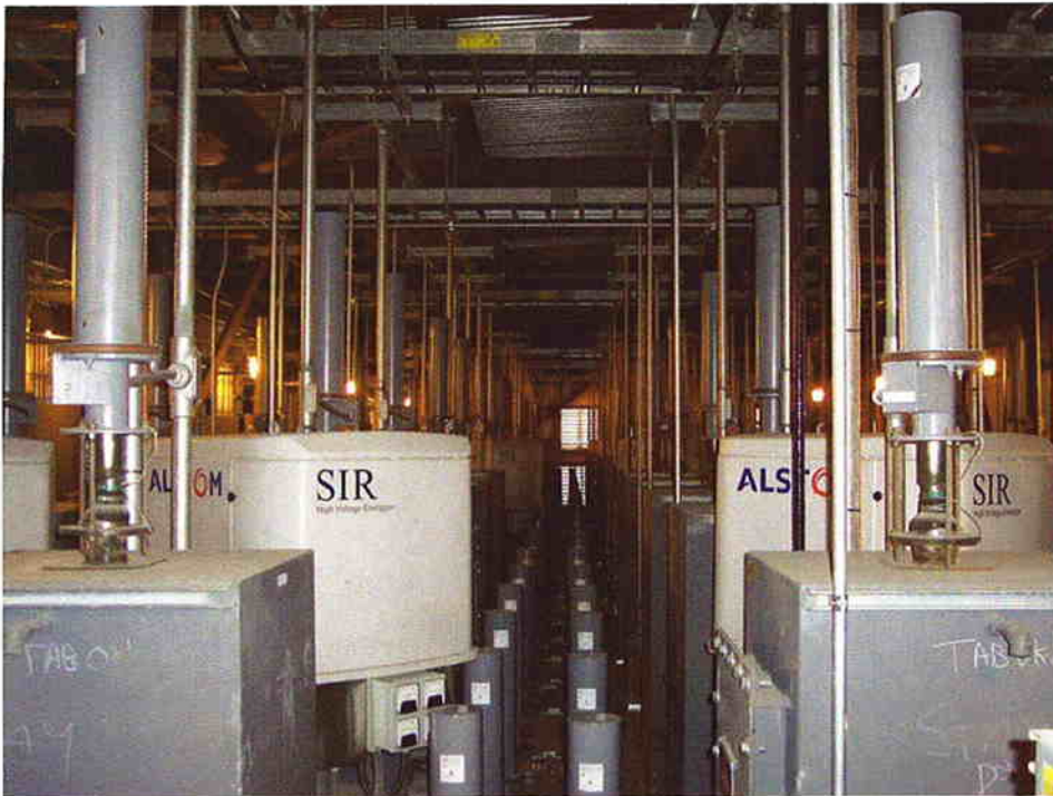
An electrostatic precipitator (ESP) is a particulate collection device that removes particles from a flowing gas using the force of an induced electrostatic charge.
