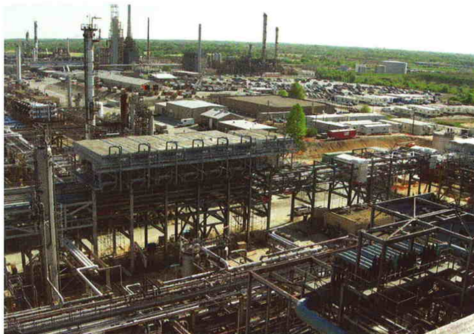
Project work completed by Nooter Construction
